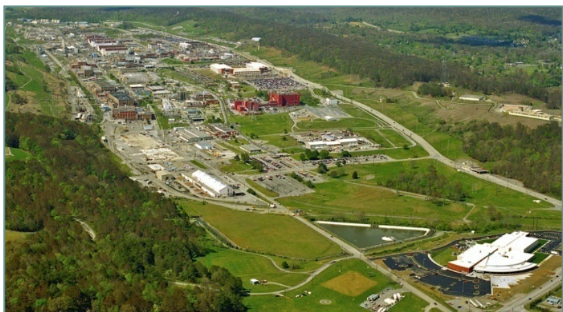
Aerial photo of the Y-12 National Security Complex, in Oak Ridge, Tennessee. Y-12 plays a vital role in the Department of Energy's Nuclear Security Enterprise helping ensure a safe and reliable U.S. nuclear weapons deterrent. Y-12 also retrieves and stores nuclear materials, fuels the nation's naval reactors and performs complementary work for other government and private-sector entities. Y-12 photo.
